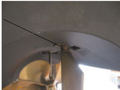
Figure 7- Completed Rudder Modifications
